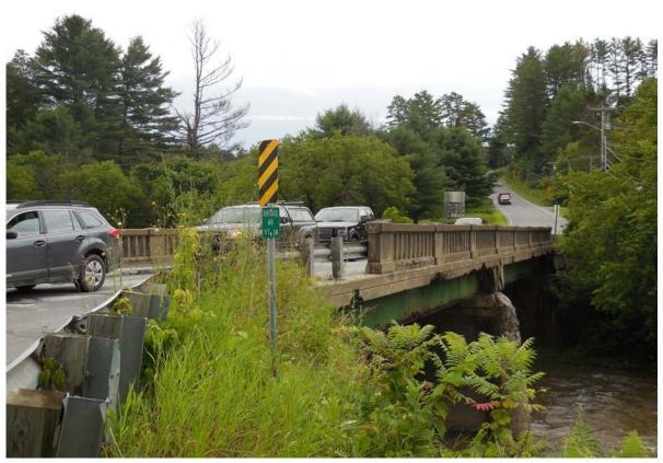
The Vermont Agency of Transportation (VTrans) is holding a Public Information Meeting to update and respond to input from the previous meeting, on the plans to replace the bridge and reconstruct the intersection at US 2/VT 14. The current plan is to replace the aging structure, add turning lanes and signalize the intersection.
