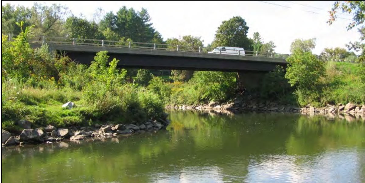
Figure 12: Route 2 Bridge with difficult alignment, R22-A. Photo credit: Johnson Company
