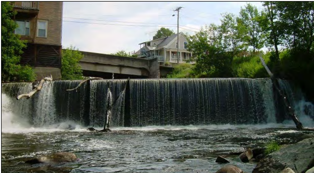
Figure 3: Dam in Plainfield Village on Reach R27-A.
