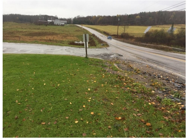
A gravel wetland is proposed in the greenspace across from the sign (pictured above). A driveway culvert will be added to the right of the sign to direct drainage to the practice.
