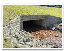
DeWolfe performed civil design for an 85 foot long pre-cast concrete box culvert replacing an existing 8' diameter corrugated metal pipe under Beanville Road. The culvert is approximately 20' below the road surface. The design included slope stabilization and a 48" bypass culvert. A Vermont Stream Alteration General Permit was obtained for the project. DeWolfe provided construction administration in challenging soil conditions, including addressing liquefying soils at the culvert foundations.
