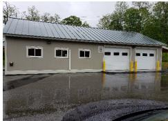
State of Vermont Department of Buildings and General Services, EHD and DEA designed and provided construction documents for a new maintenance facility for the Newport Prison. The building is approximately 2,800 sf and includes office space and garage space with a mezzanine for mechanical equipment. It is designed to meet the State's requirement for achieving 30% above the already stringent Vermont Commercial Energy Code. The project is awaiting funding for construction.
